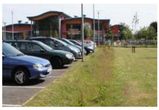
Figure 17: Shallow car park swale with very high infiltration in Bushloe High School in Wigston, Leicestershire (Image credit: DSA Environment + Design)
