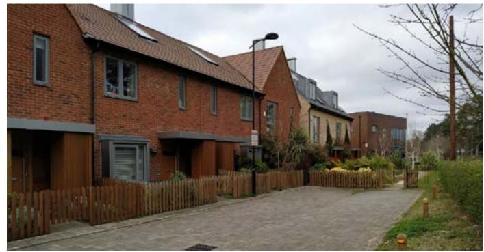
Figure 50: Integrated bin storage built into the front porch of new homes. This is an optimal solution.
